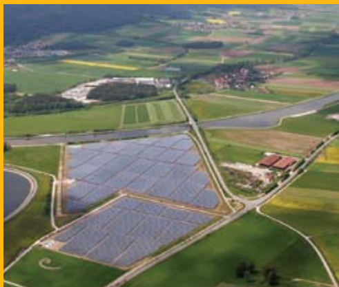
Bavaria Solar Park - 10 MW - Bavaria, Germania
